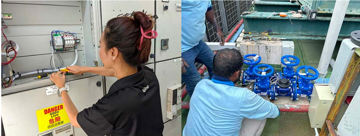
Deployment of Energy-Efficient IoT Sensors at StorHub
